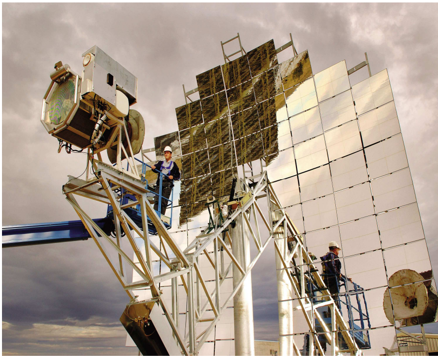
Figure 11.2.2: Stirling engine based electricity production using solar-dish concentration at Sandia National Laboratory. The system gives a solar-to-electric conversion efficiency reaching 30 percent. Each unit can produce up to 25 kilowatts of daytime power. 10
