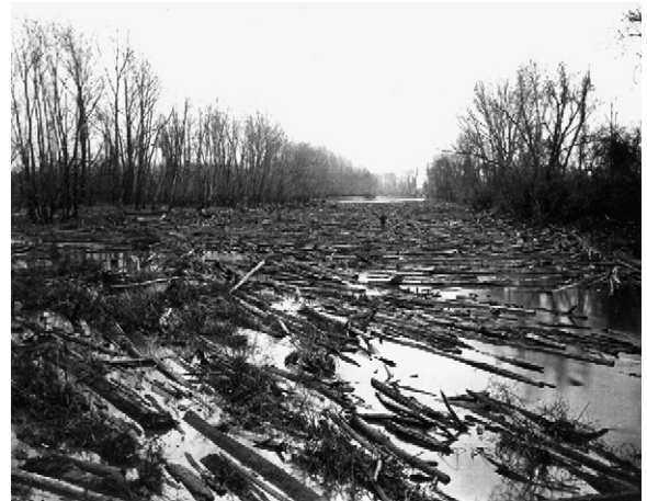
Fig. 9. Red River log jam (1873) representing thirty-four years of accumulation after the initial clearing of the channel and cessation of maintenance. Photographs by R. B. Talfor, United States Army Corps of Engineers. Photograph courtesy of Louisiana State University, Shreveport Archives.
