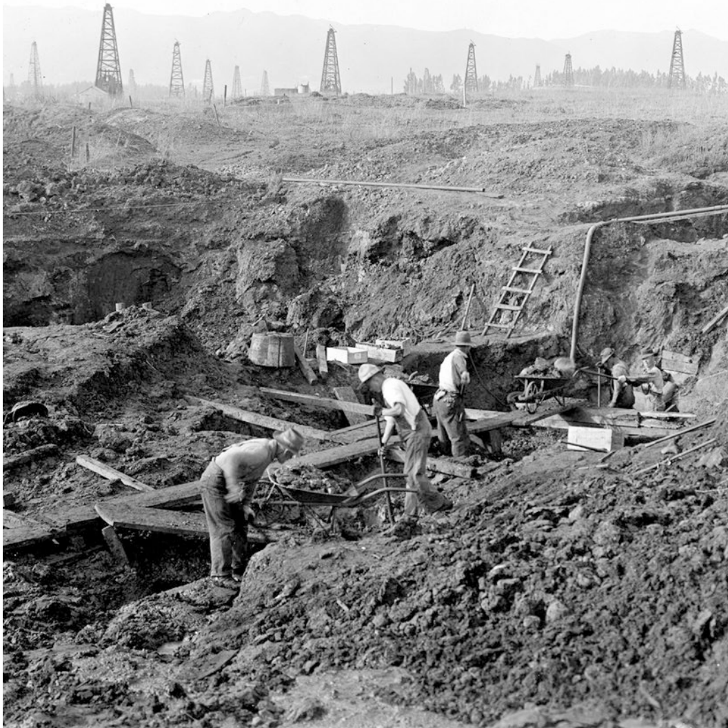
Fig. 1.8 Excavations at Rancho La Brea in the nineteenth century
